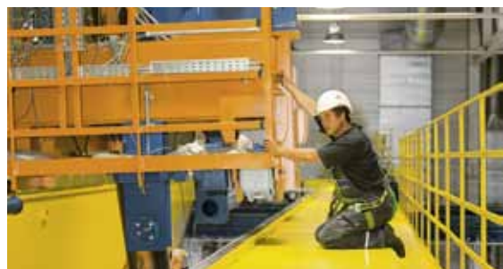
Routine work for Demag Service: precise alignment of the open-winch crab
