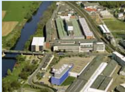
EUR 14 million has been invested in modernisation of the production infrastructure.
