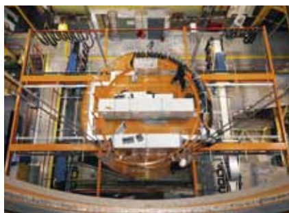
Pre-assembly work on an intermediate platform
