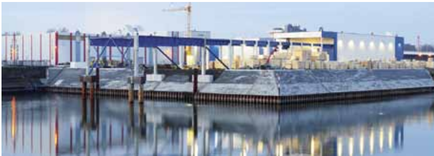
dpl packing building: the crane runway extends into the harbour basin
