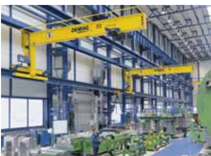
Two wall-travelling cranes used for transporting and positioning material
