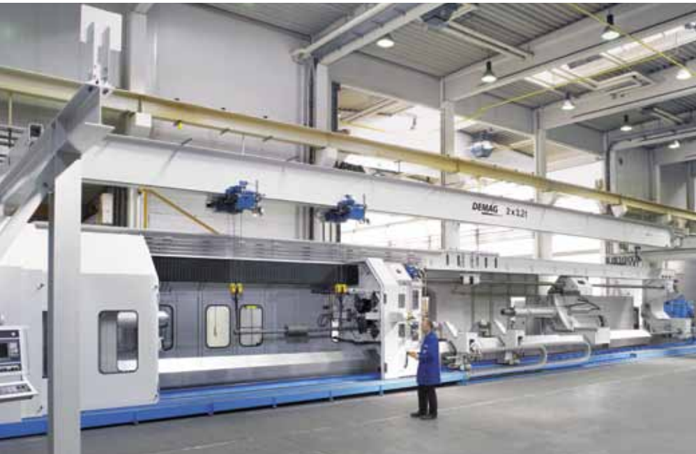
EKKE and two 3.2 t wire rope hoists serving the longest spinning machine in the world
