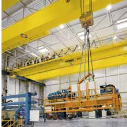
A second bridge crane lends support during delivery of the crab
